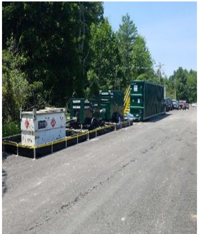
Fig 4: College Brook bypass tank and pumps arrived on site. Viewing southwest. (7-09-19).
