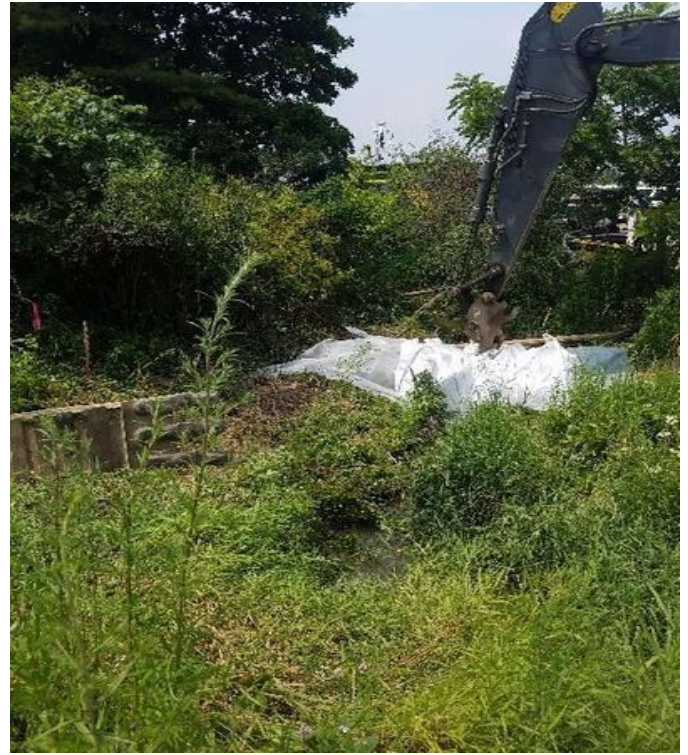
Fig 10: McCourt placing sand bags for coffer dam. Viewing west. (7-10-19).
