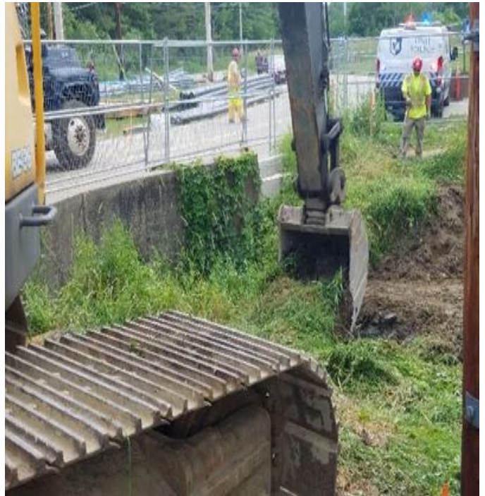
Fig 12: McCourt removing the topsoil and vegetation to re-use during remediation. Viewing south. (7-10-19).
