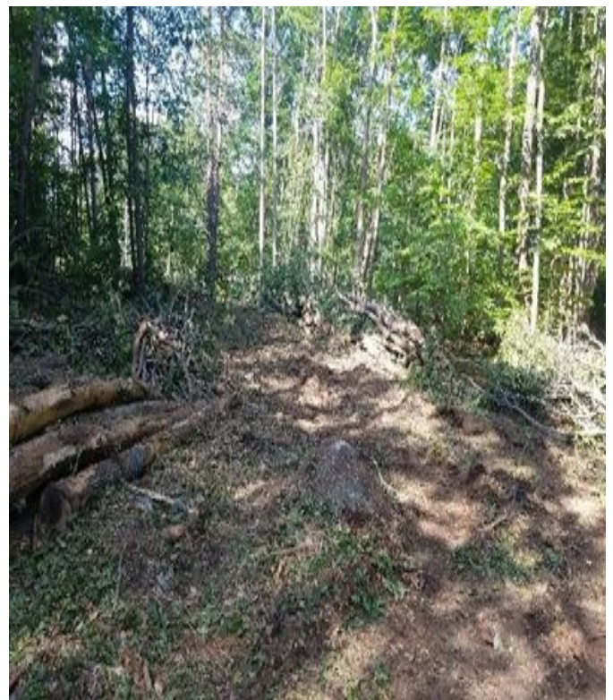
Fig 8: Access Rd off of Mill Rd tree clearing. Viewing north. (7-09-19).
