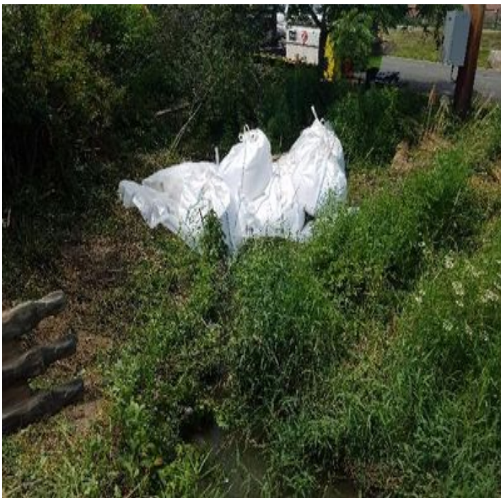
Fig 11: Completed coffer dam in College Brook. Viewing west. (7-10-19).
