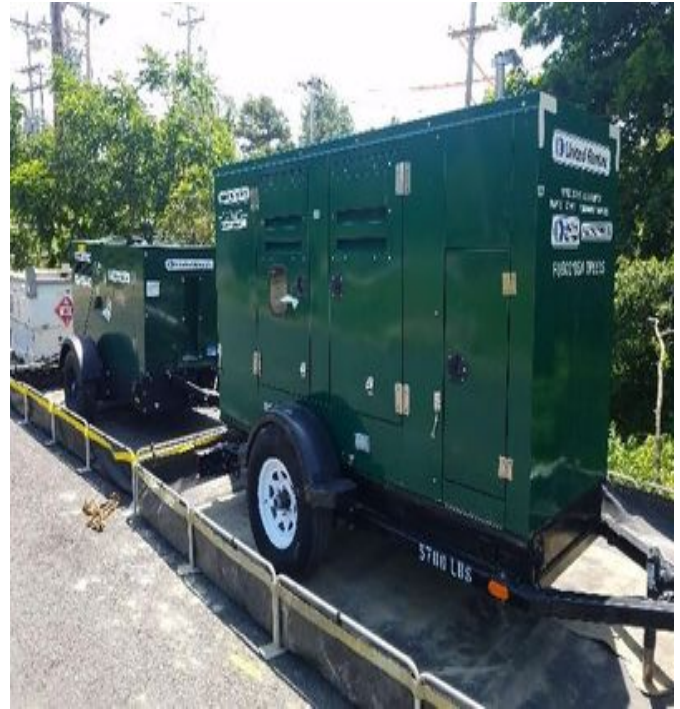
Fig 6: Pumps for College Brook bypass. Viewing south. (9-09-19).
