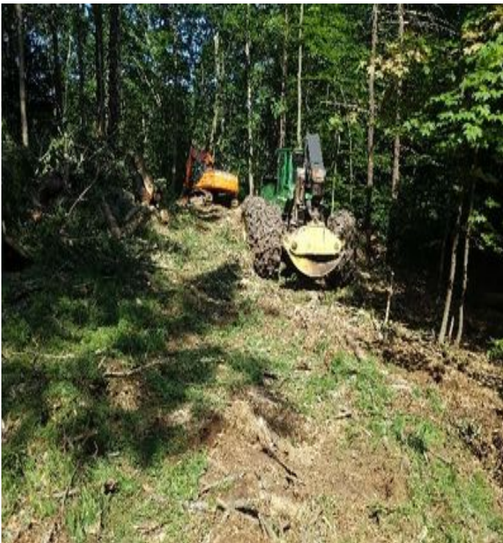
Fig 7: Access Rd off of Mill Rd tree clearing. Viewing north. (7-09-19).
