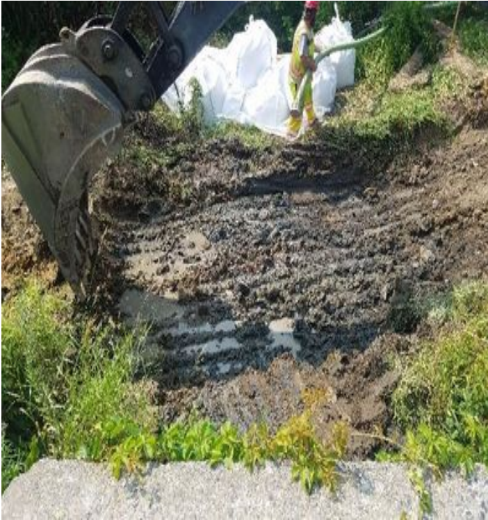
Fig 13: McCourt excavating College Brook. Viewing west. (7-10-19).
