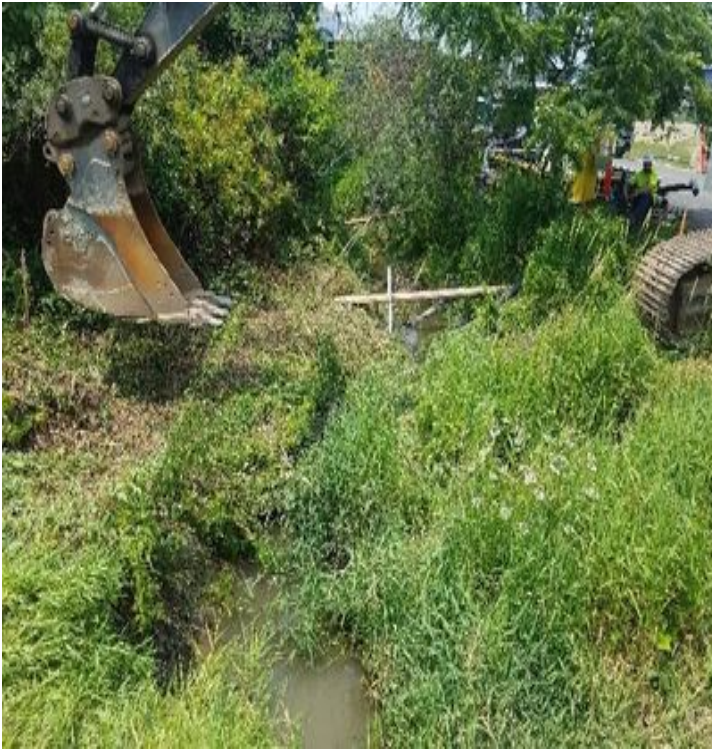
Fig 9: McCourt prepping College Brook before placing the coffer dam. Viewing west. (7-10-19).
